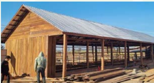
Figure 26 | New roof on school building
