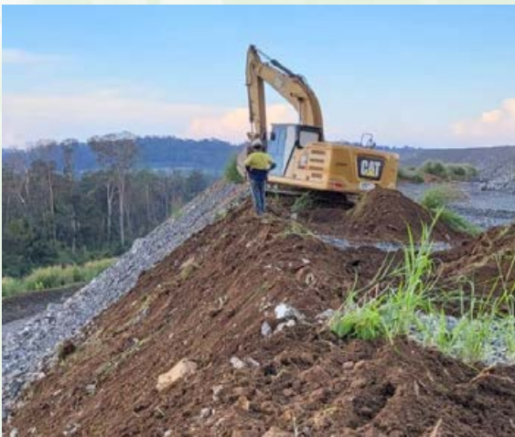
Figure 18 | Okvau batter/berm trial
