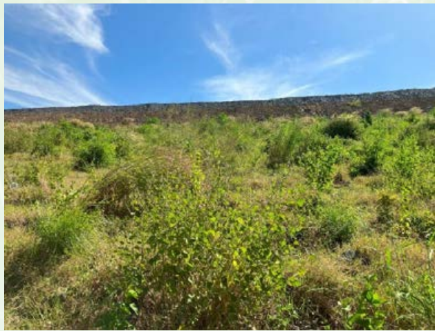
Figure 19 | Okvau waste rock dump under rehabilitation
