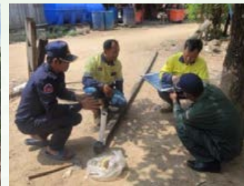
Figure 28 | Installing roadside lighting
