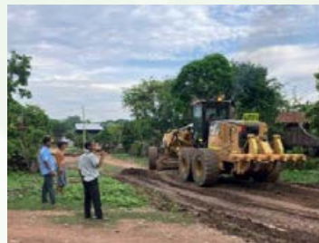
Figure 27 | Village road upgrades
