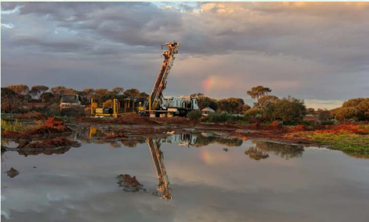
Figure 23 | Drill rig at Dingo Range Gold Project
