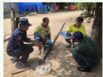
Figure 47 | Installing roadside lighting
