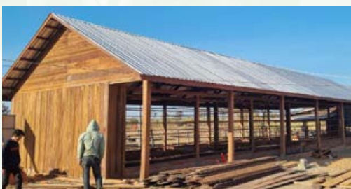
Figure 45 | New roof on school building
