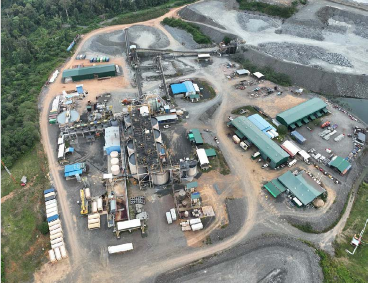
Figure 7 | Okvau Processing Plant
