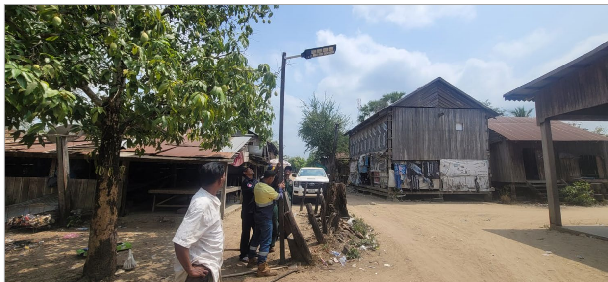
Figure 26 | Village police and Company staff installing roadside solar lighting
