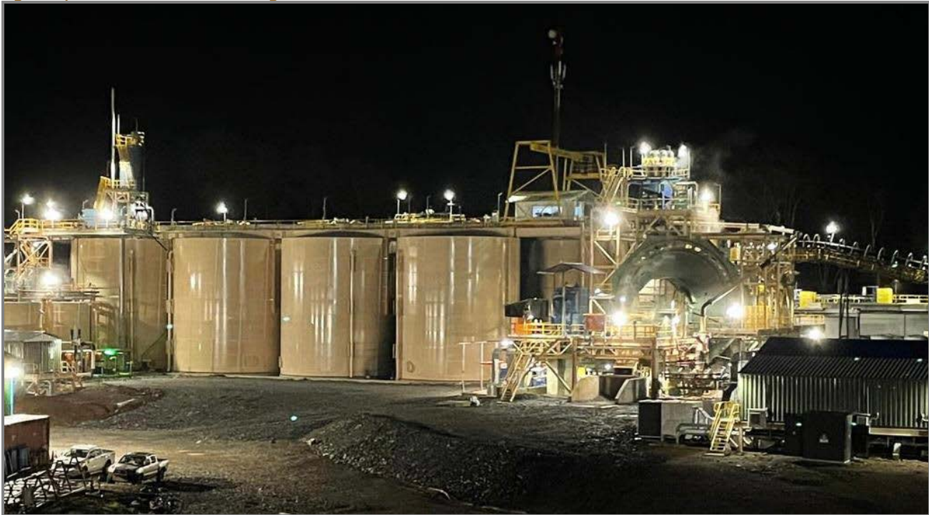
Figure 3 | Okvau Gold Mine Processing Plant
