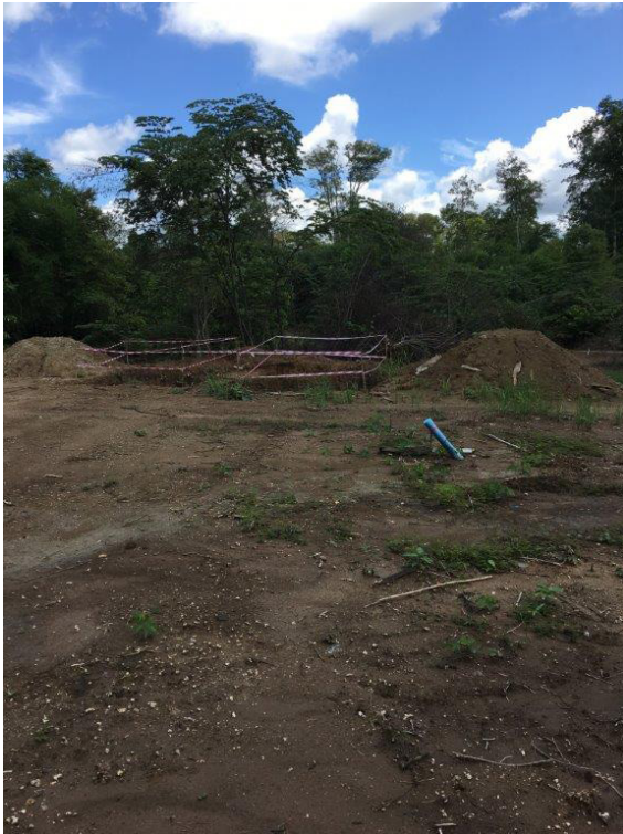
Figure 6: Drill Pad ready at Samnang
