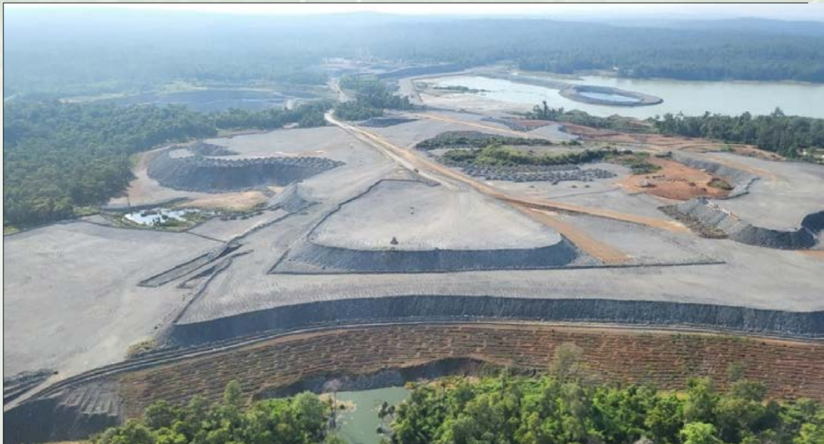
Figure 1 | Okvau’s tailings dam and waste dumps
