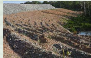
Figure 7 | Rehabilitated batter on waste dump
